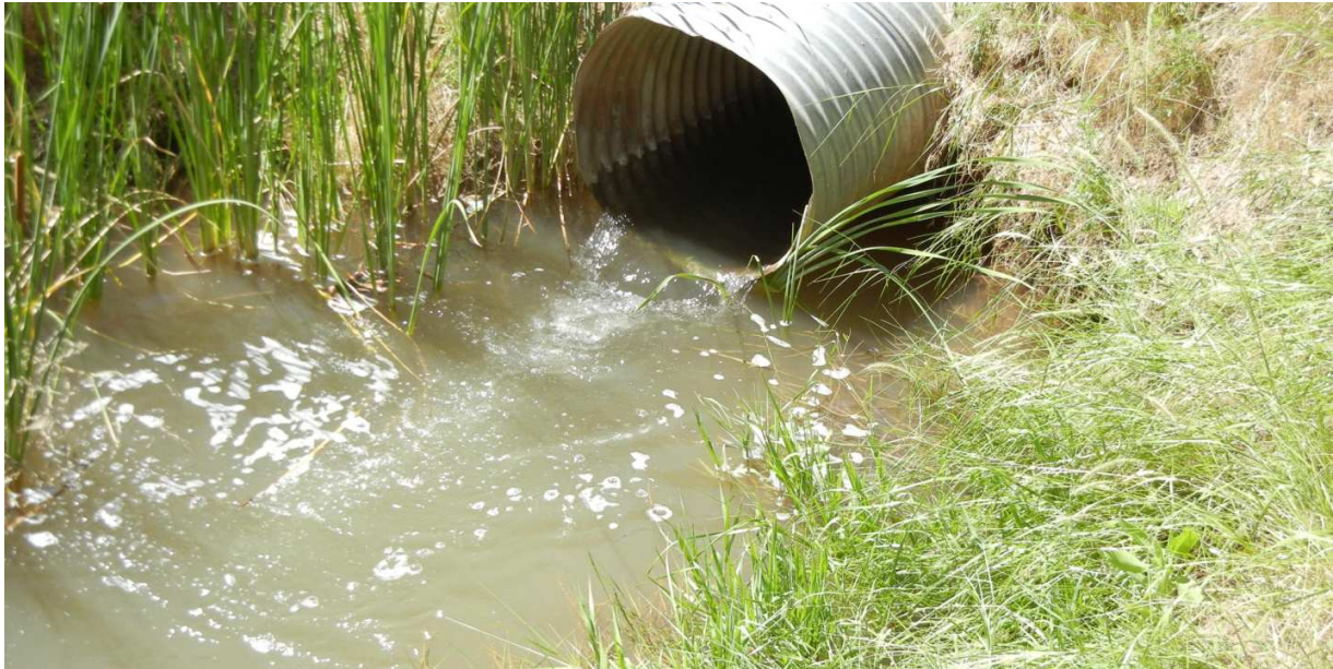
A gravity flow surface water diversion ditch from the Verde River.
